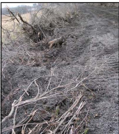
Left Photo)View west from Nelson Road toward Harp Road—note tree and brush cuttings, plus base material from old rail-bed, dumped into adjacent drainage ditch.
