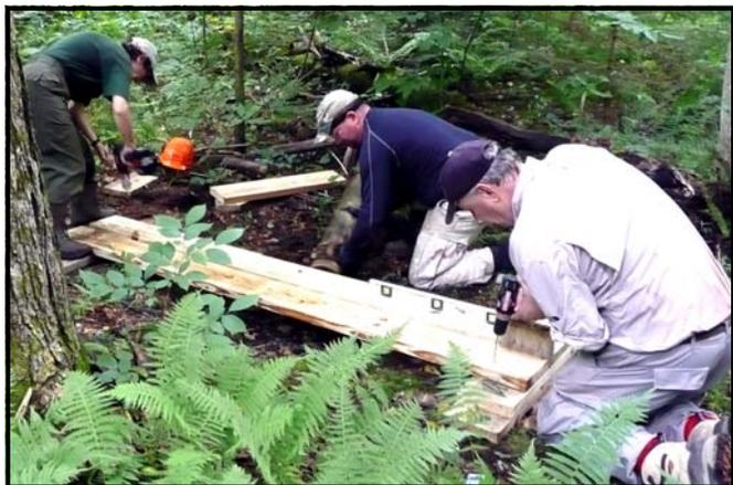
The total area spanned as needed approximated 150+ feet. The expected long service life of these puncheons, sometimes termed bog bridges, will confine foot traffic to a single path—a good outcome.
